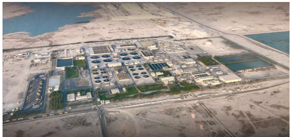
Sewage treatment plant of Doha West - Treatment of urban wastewater - operated by Suez - Qatar
